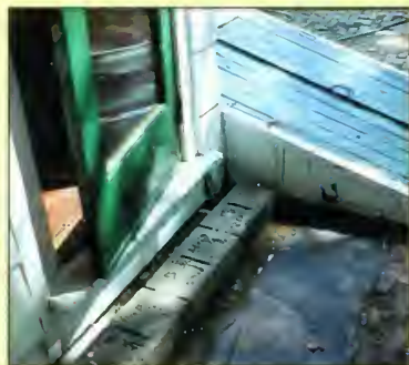
Many older homes have outdoor access to the basement—often double wood doors that lead to a steep concrete stairwell. For safety's sake, keep the doors locked. Also, replace warped or rotting doors so that if kids play on them, there's no chance that they'll fall through.
